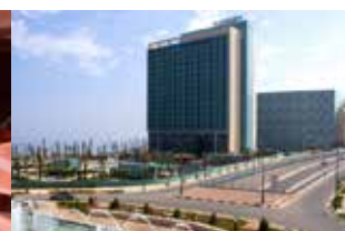
Vista exterior Exterior view
